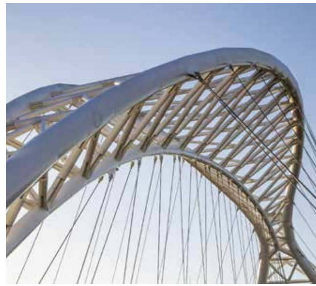
Stahlbau Structural steelwork
